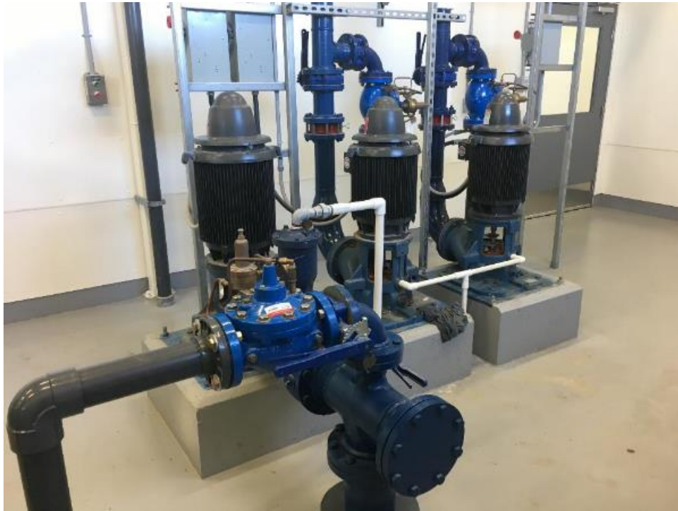
Transfer pumps and backwash pump.
