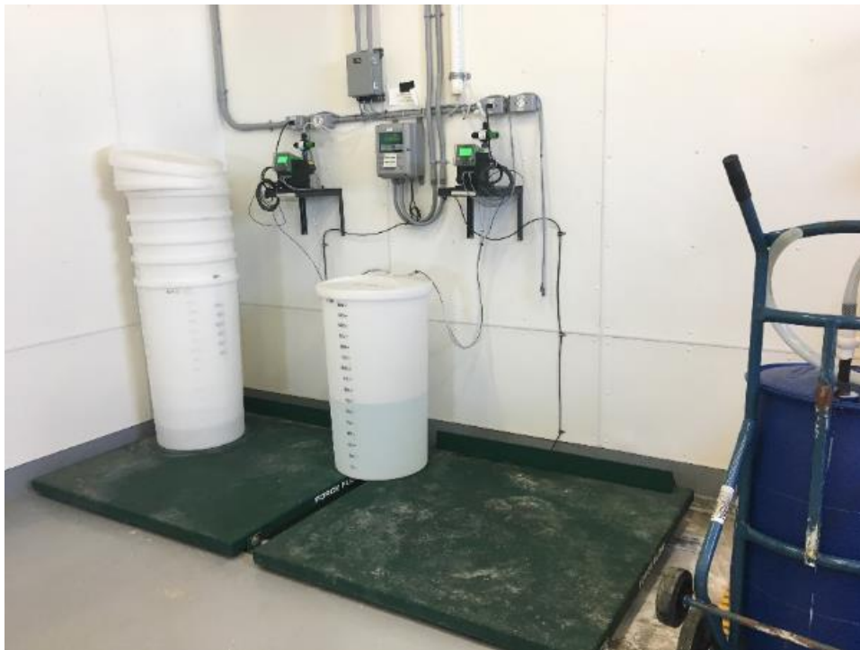
Chemical feed set-up.
