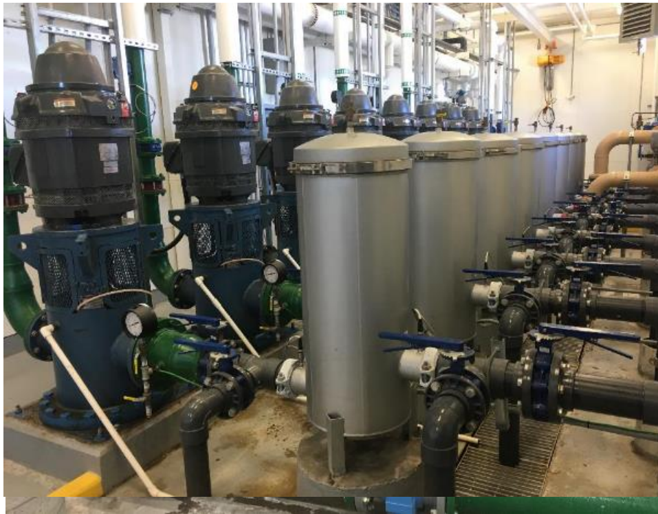
Booster pumps and pre-filters.
