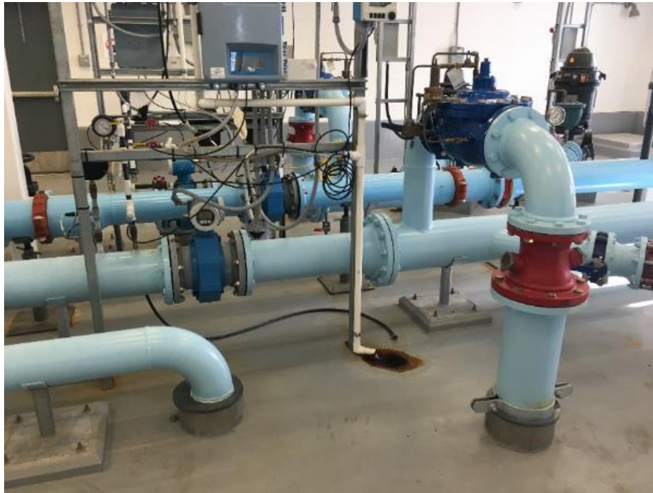
Distribution piping, PRV valve.
