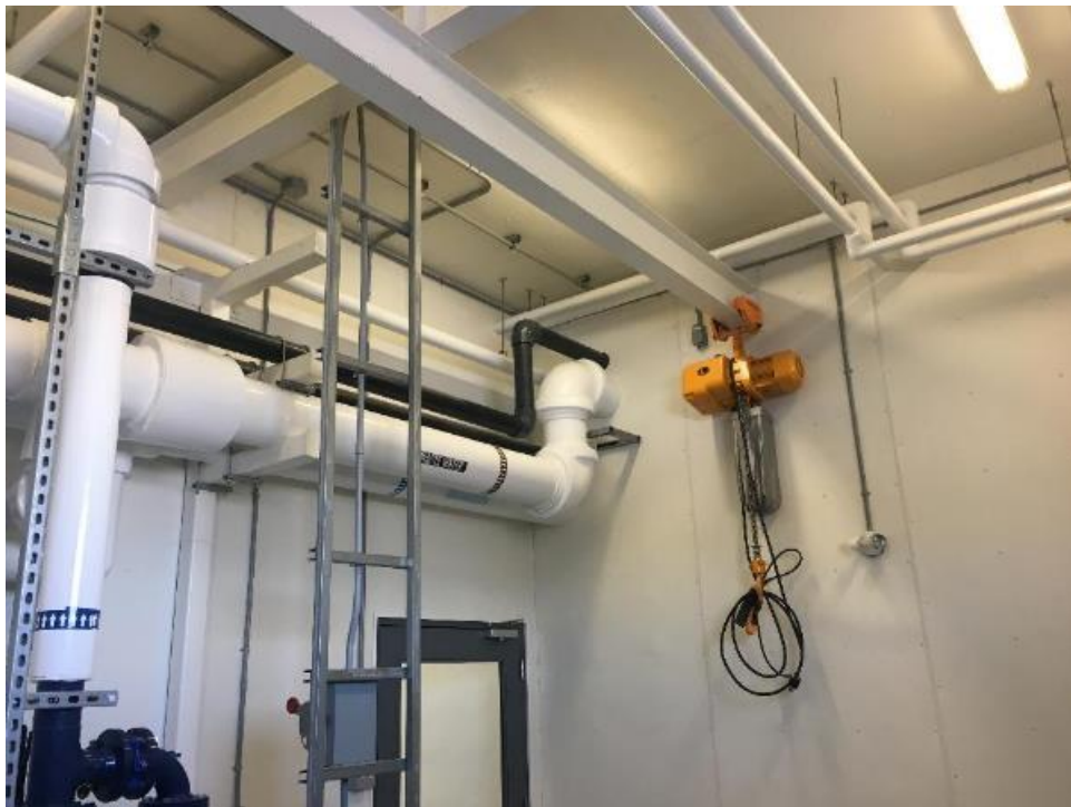
Electric hoist in booster pump room.
