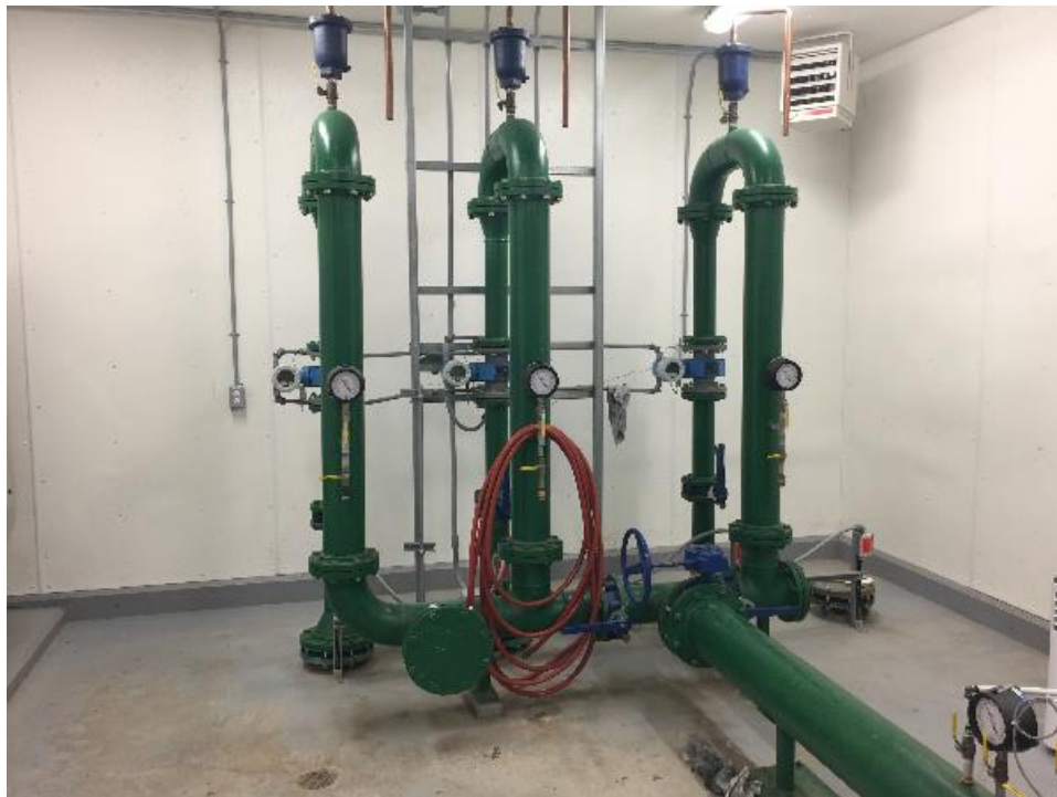
Raw water main header from each well.
