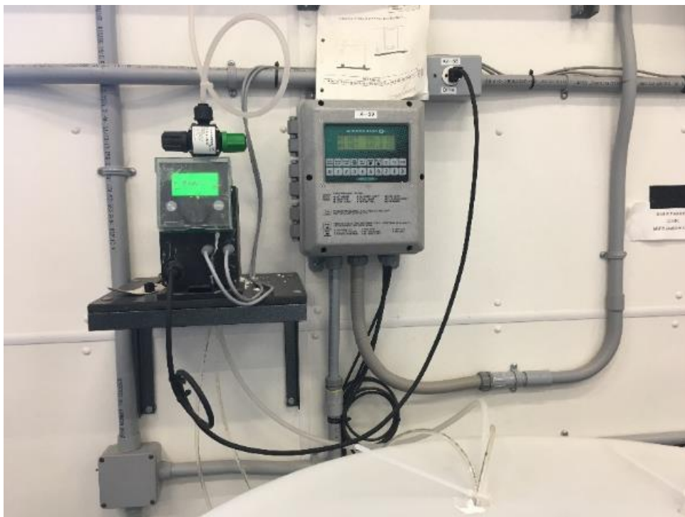
Chemical feed pump and weigh scale interface.
