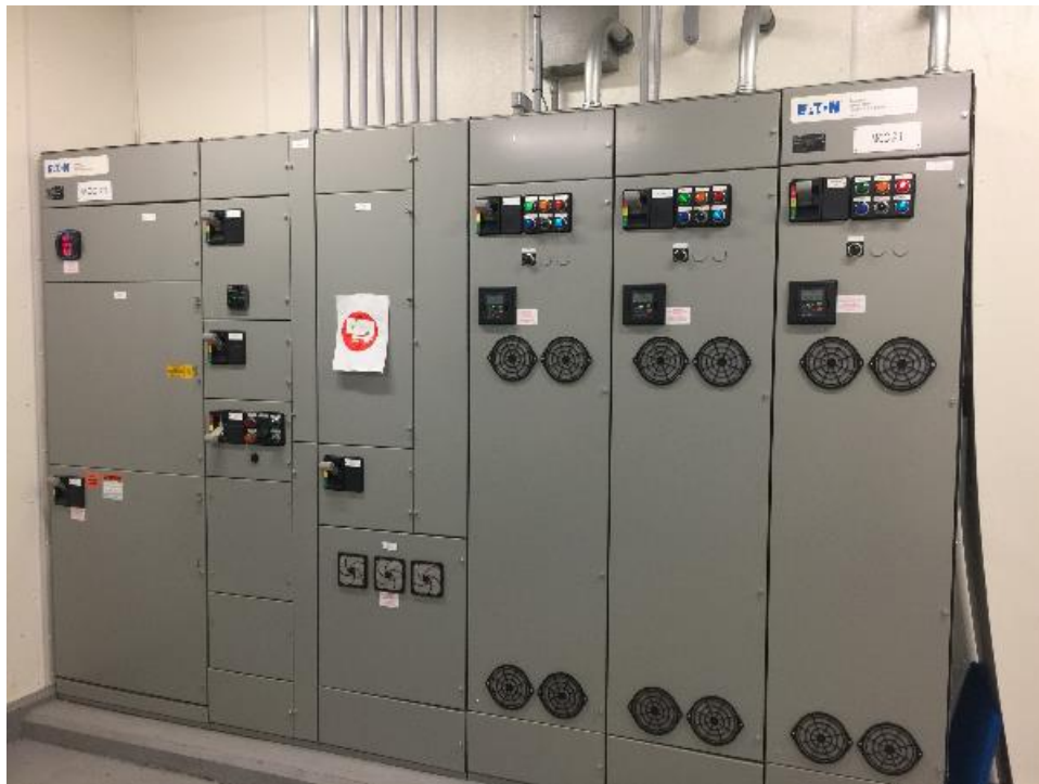
Well pumphouse electrical MCC.
