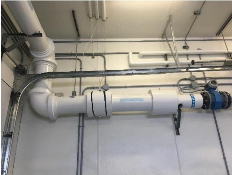
Treated water discharge to reservoir, magmeter.
