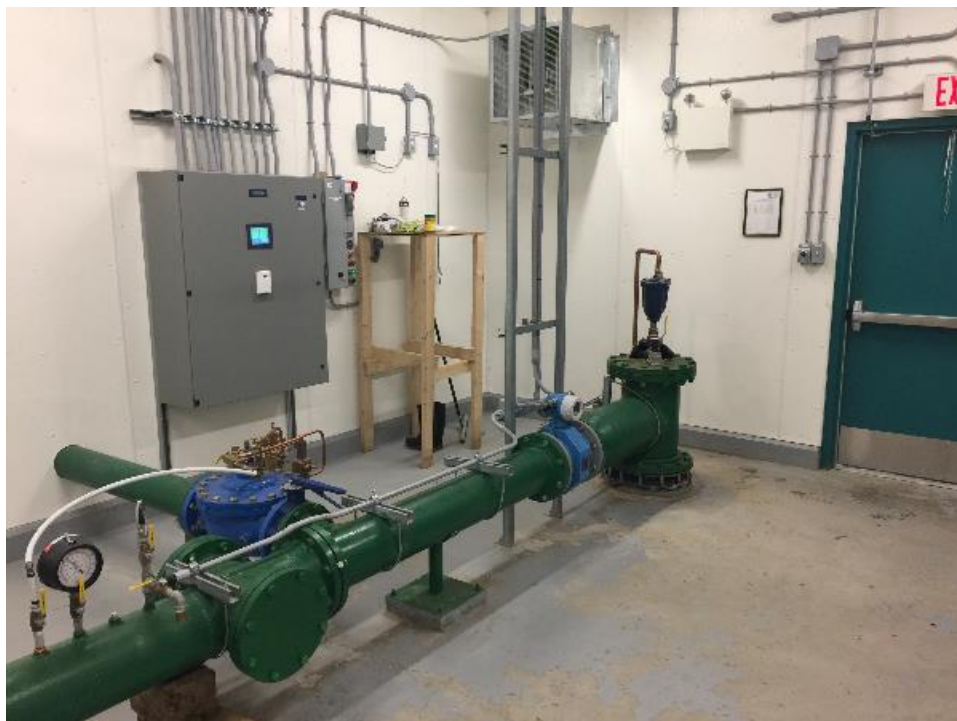
Raw water main header, PRV, and flow meter.
