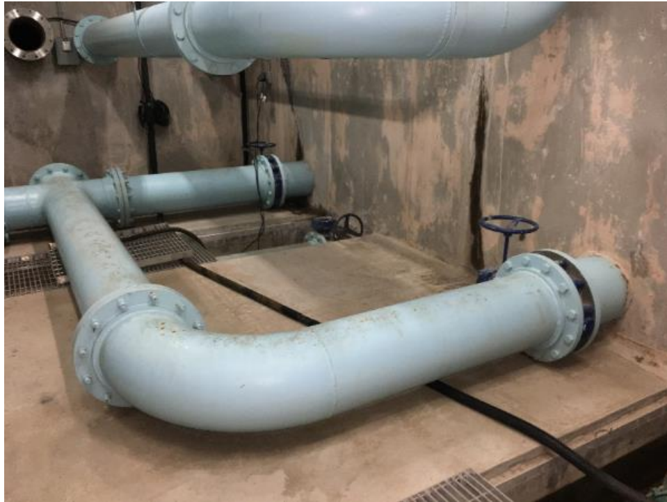
Distribution piping in valve chamber.
