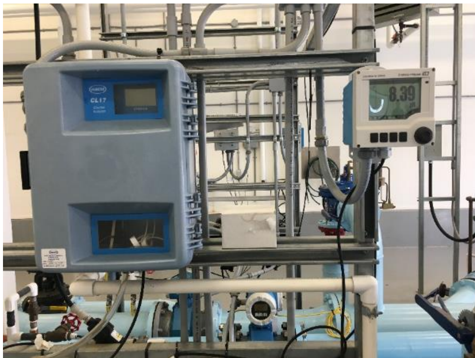
Distribution header, magmeter, pH meter, and chlorine analyzer.
