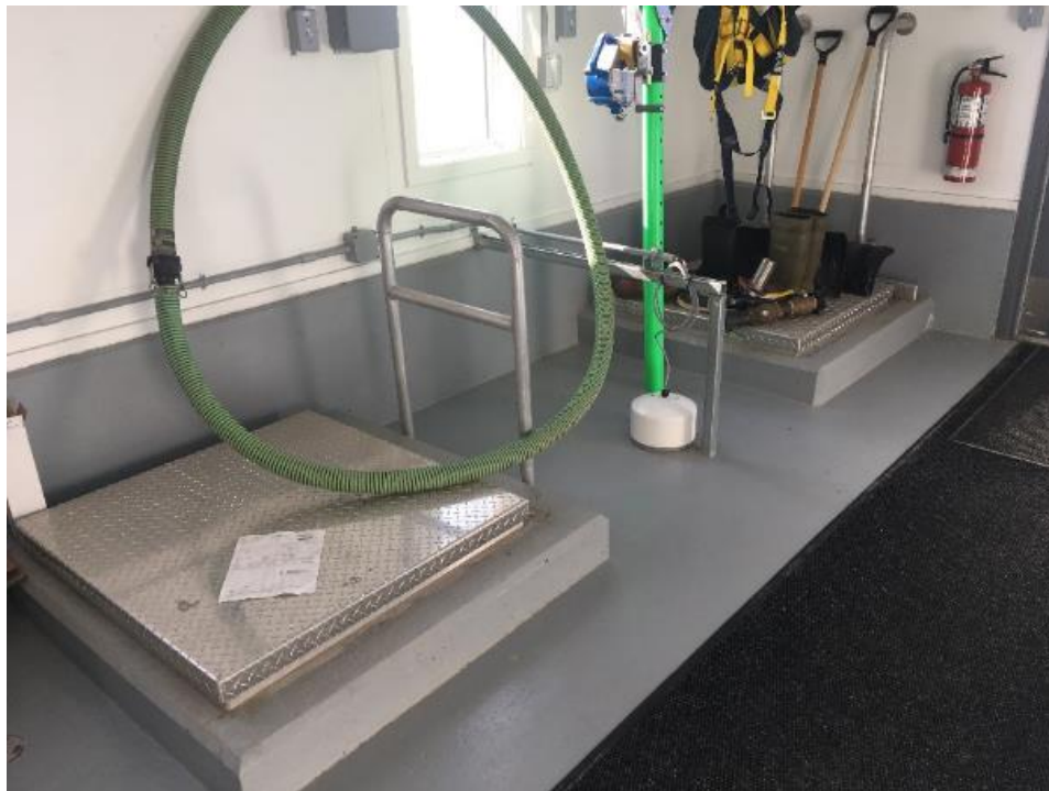
Reservoir access hatches and level sensor.
