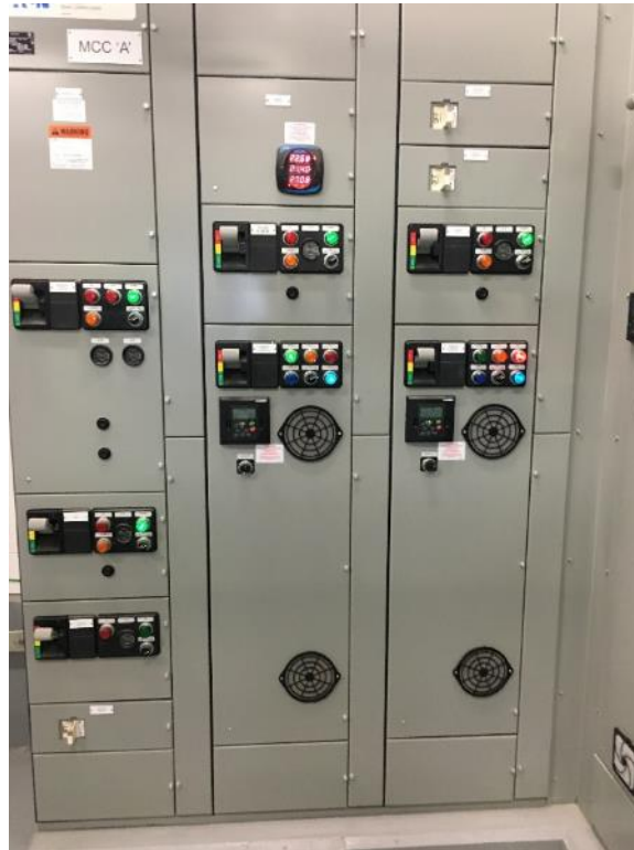
Variable frequency drives in electrical room.
