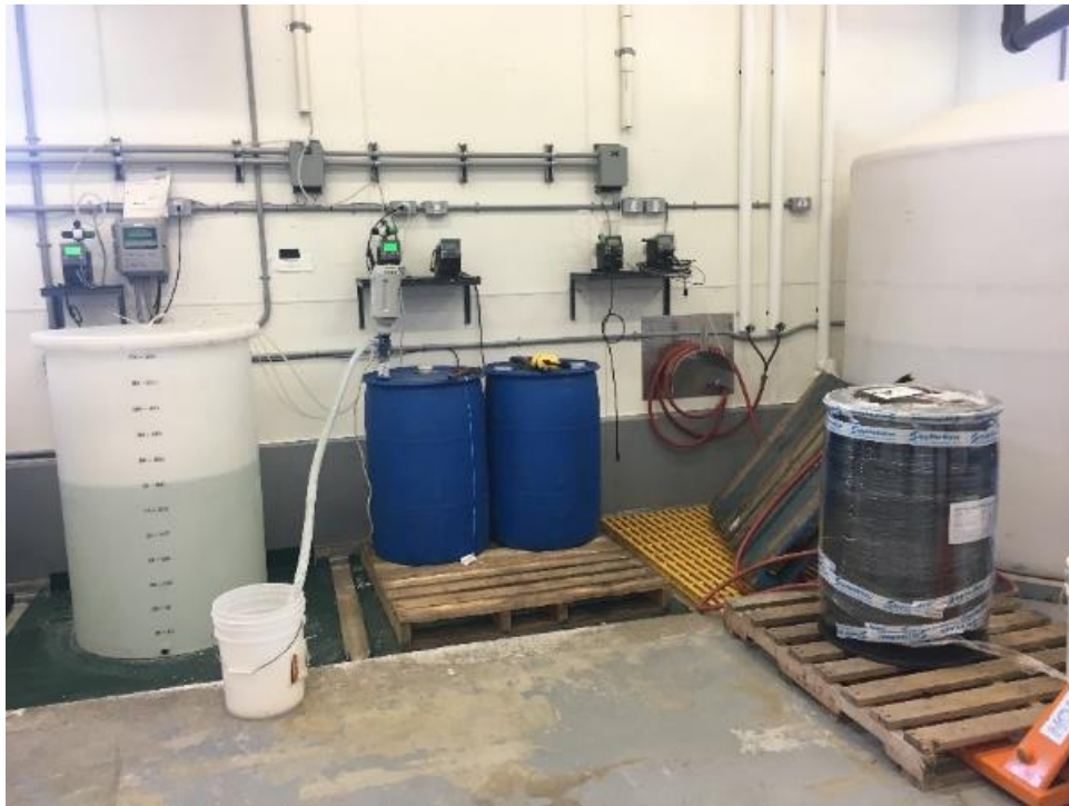
Chemical feed, in-floor scales, feed pumps.
