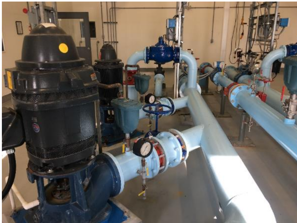
Distribution pumps and header.
