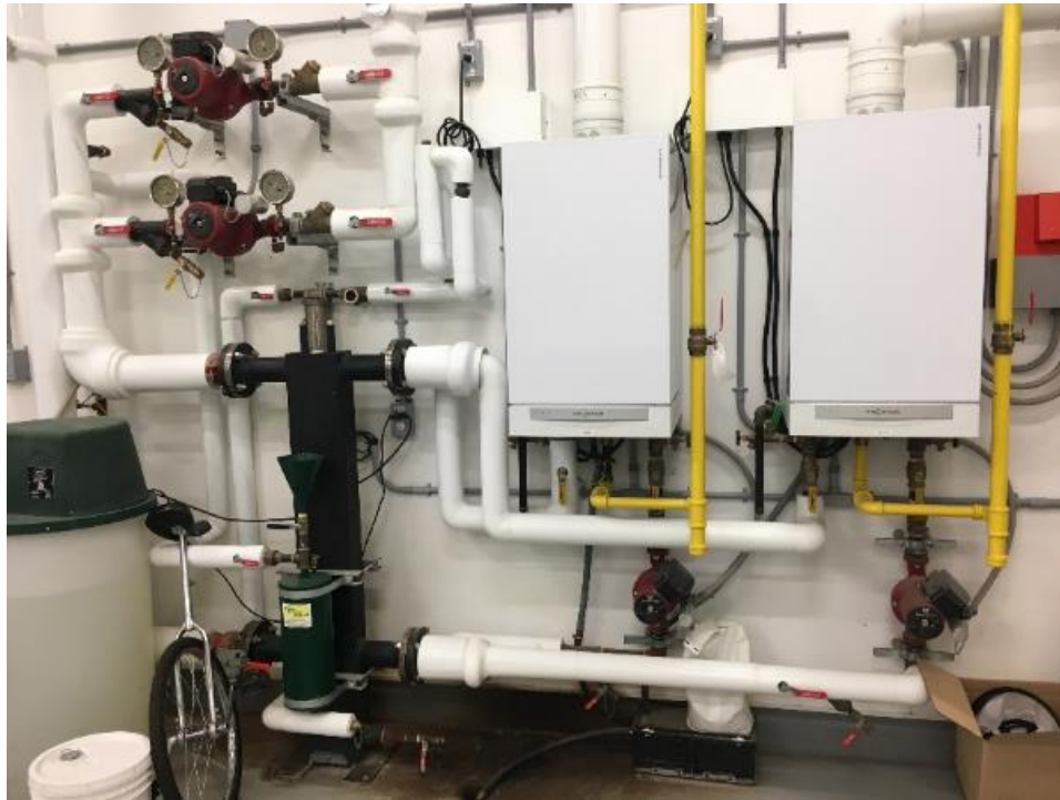
Natural gas boilers (heating system).
