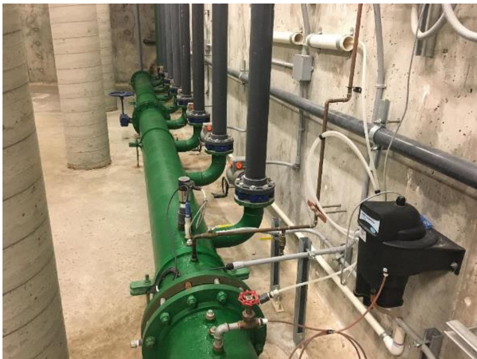
Raw water main entering WTP, turbidity meter.
