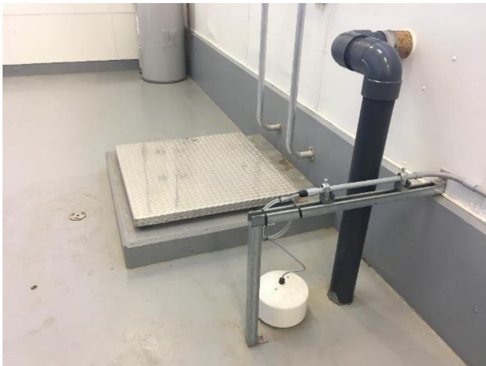
Flushing chamber access hatch and level sensor.
