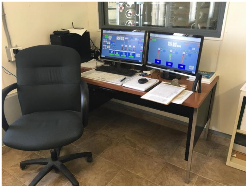
Operator PLC control interface.
