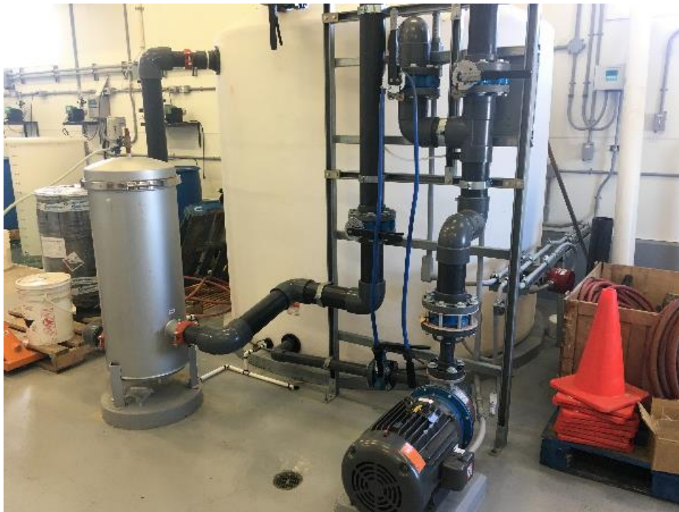
Clean-In-Place tank, pre-filter, and pump.
