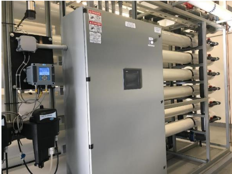
Membrane treatment unit controller, turbidimeter.
