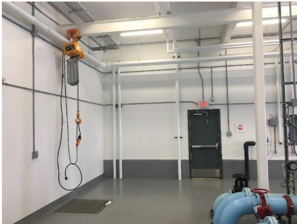
Overhead electric hoist in distribution pump room.
