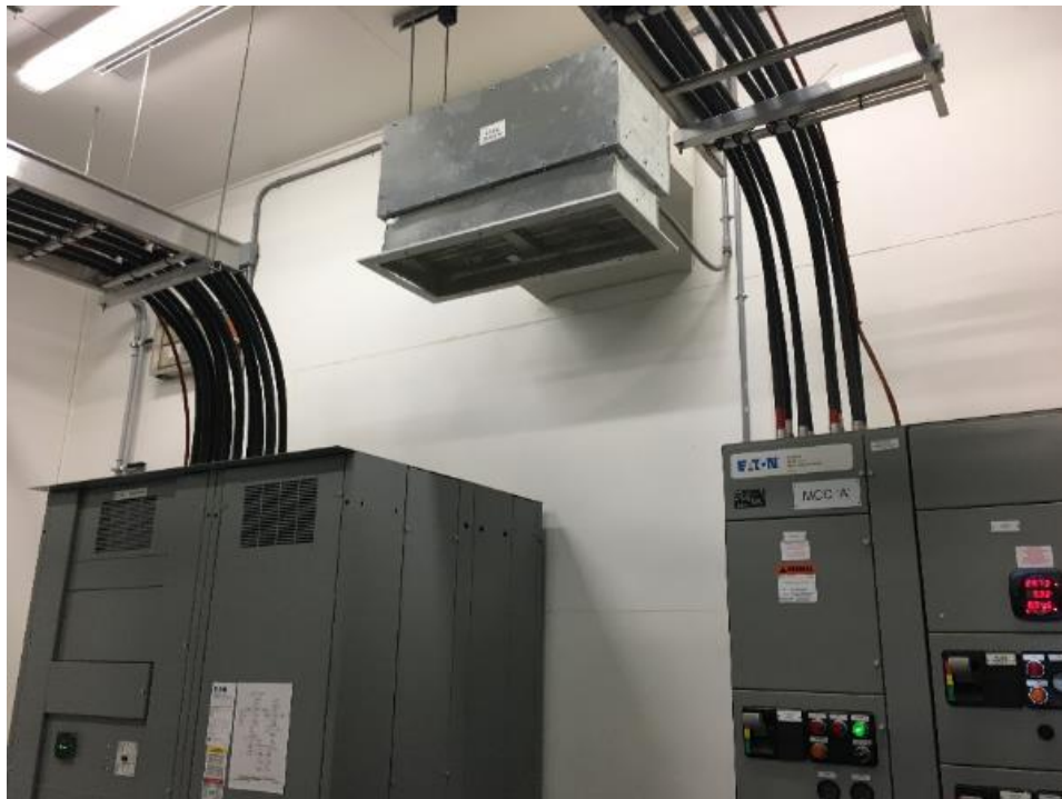
Electrical room ventilation equipment.
