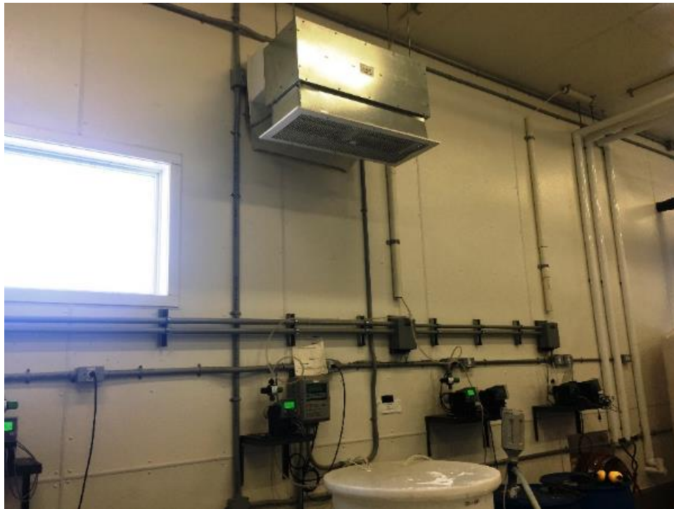
Chemical feed room ventilation.
